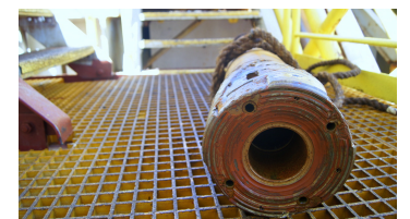
The bottom of the damaged drill bit that is missing all of its drill cones. Photo by Amy West
